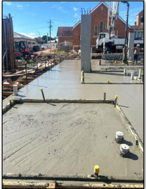
Pouring the slab for the new build
