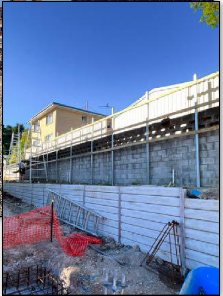
New retaining wall and fence on the southern boundary
