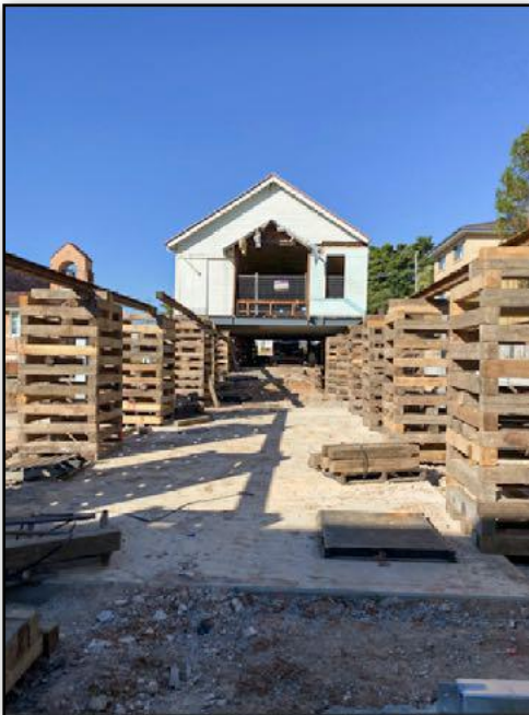
Preparing to move the old hall
