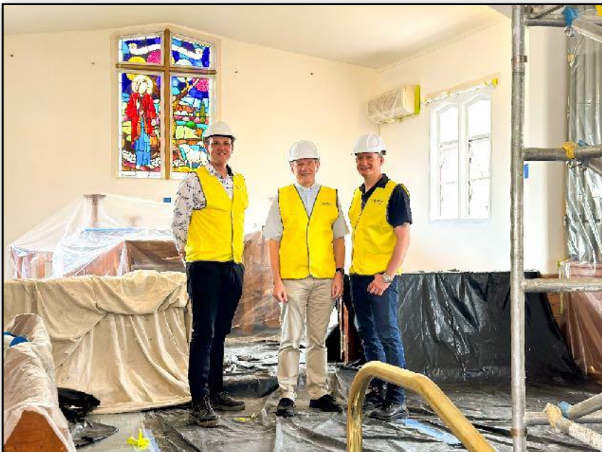
Painting in progress within the church
